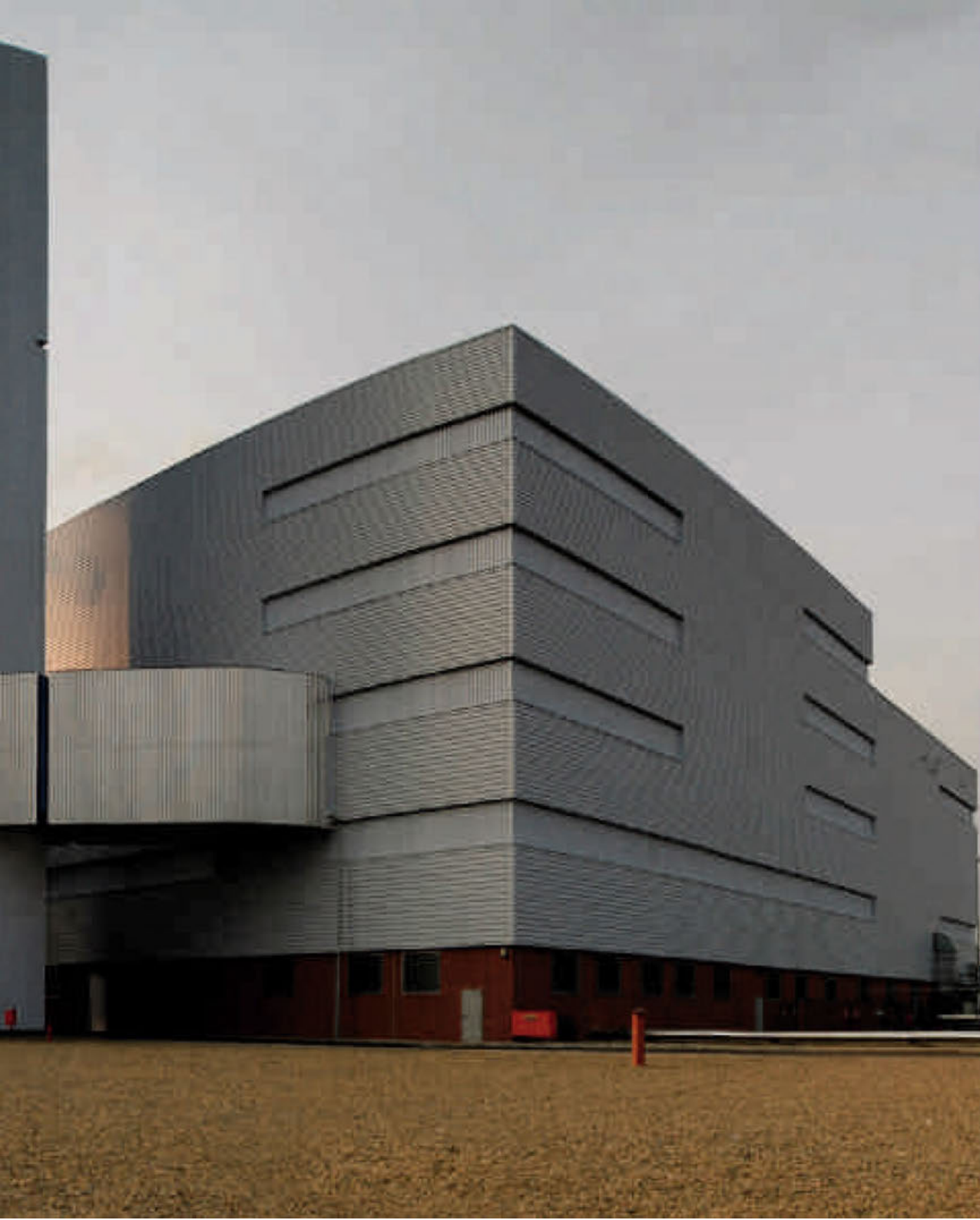
Livorno Ferraris Power Plant - Italy
