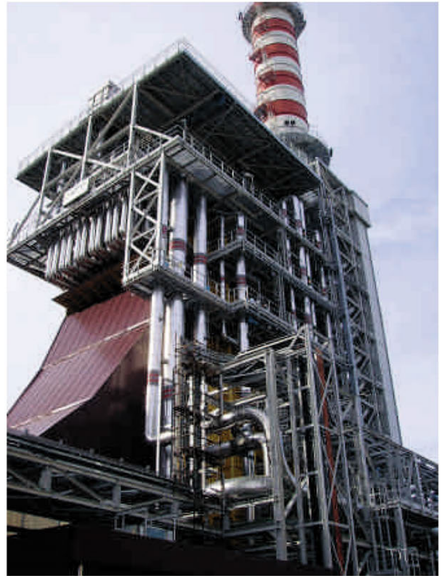
Termini Imerese Power Plant - Italy
