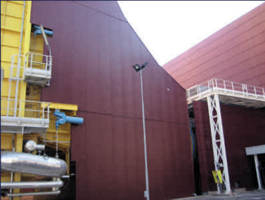
Termini Imerese Power Plant - Italy
