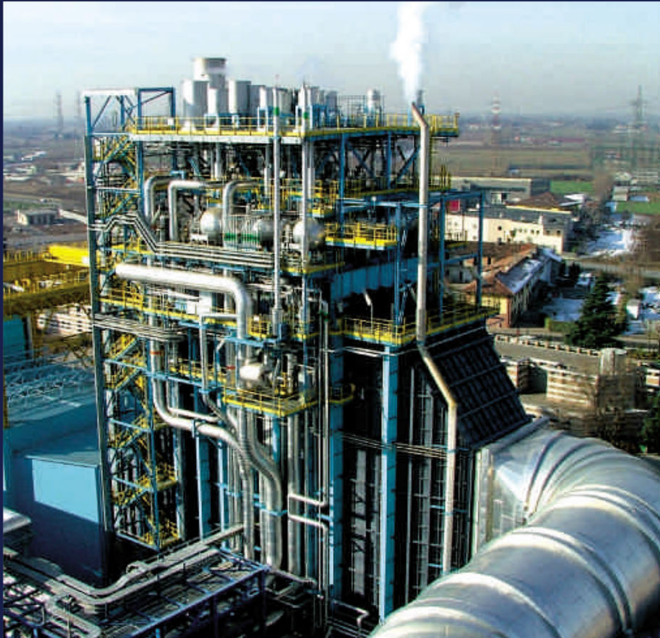
Cassano D'Adda GR6 Power Plant -Italy
